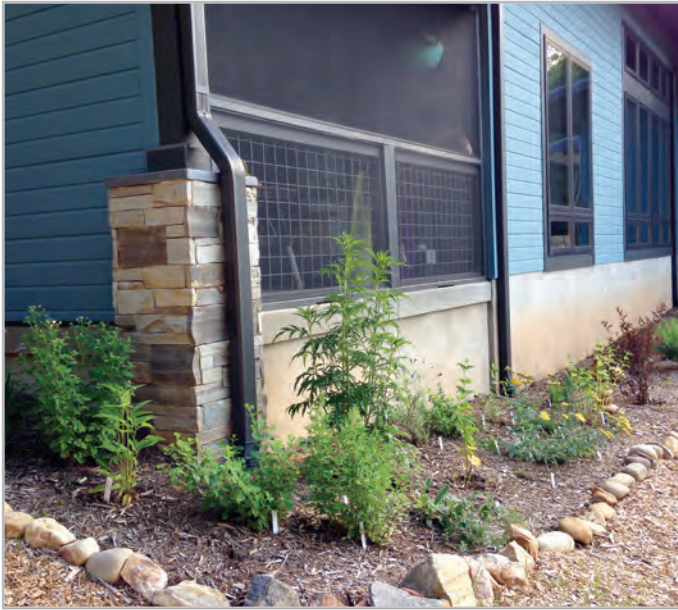
A newly established kitchen herb garden sits below a screened porch at a house built as a permaculture incubator by Cardinal Point Construction, which attained Green Built Homes silver certification on the project.
